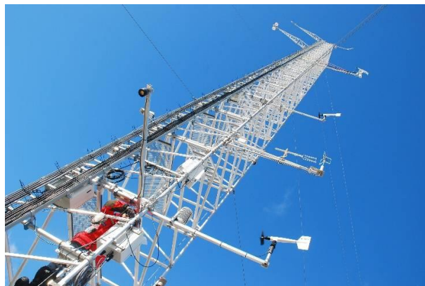
The Amundsen-Nobile Climate Change Tower during maintenance (Photo: Fabio Giardi).
