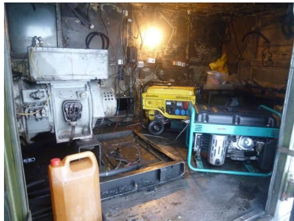
Old 10.4 kW diesel generator (left) and the new, more efficient 10.8 kW diesel generator
