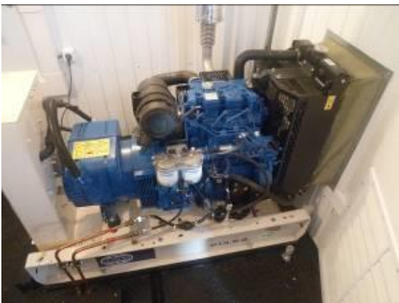
Old 10.4 kW diesel generator (left) and the new, more efficient 10.8 kW diesel generator
