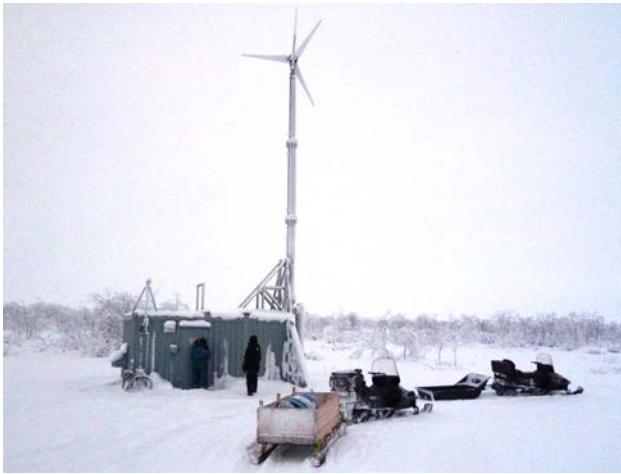
New wind-diesel plant
